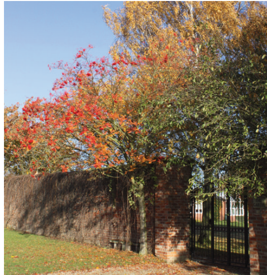
Cavity wall around The Garth, formally Stubton Hall kitchen garden
